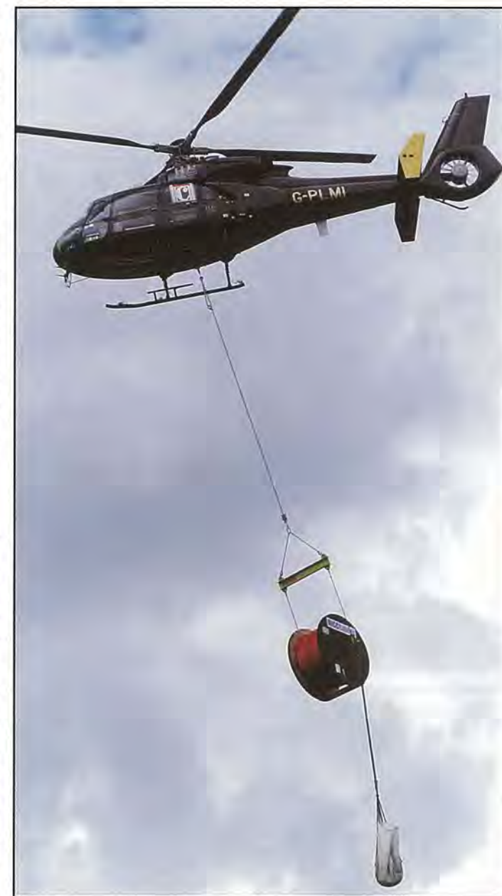
The heavy cable drums are flown up the Conwy Valley.
